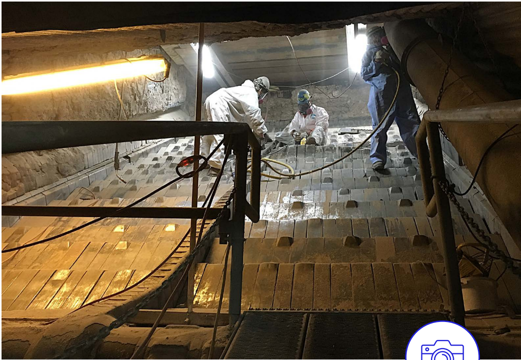
Critical outage service-stoker grate
