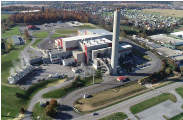
Covanta York: With superior safety and environmental performance, the York, Pennsylvania facility maintained 98.6% boiler availability and set a record for power sold in 2020.
