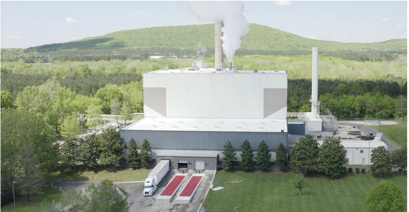
Huntsville EfW facility
