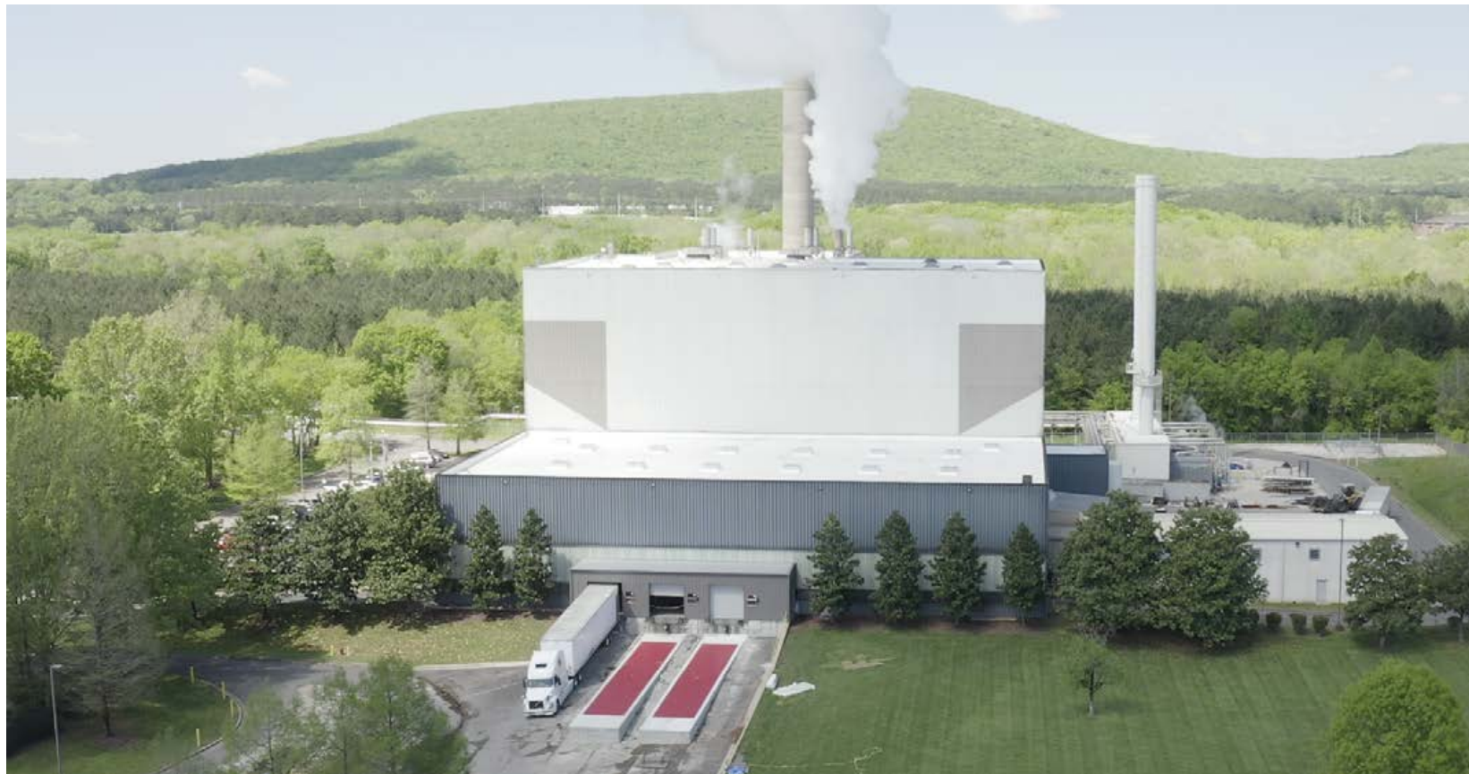
Huntsville EfW facility
