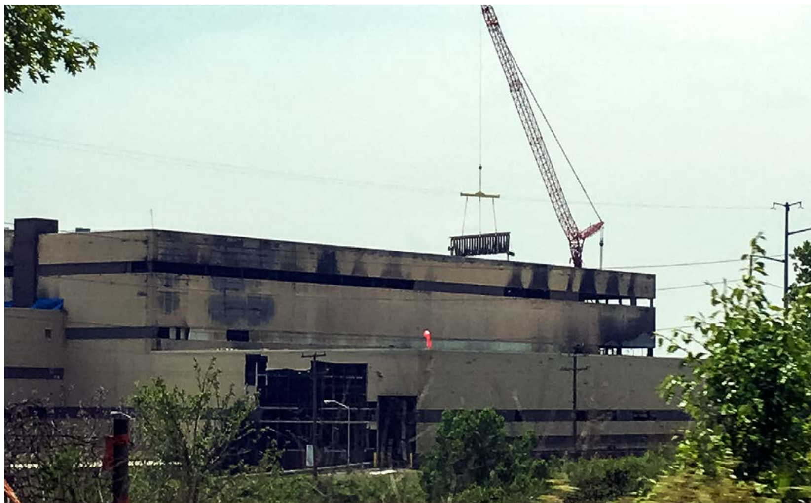
Covanta Fairfax during reconstruction
