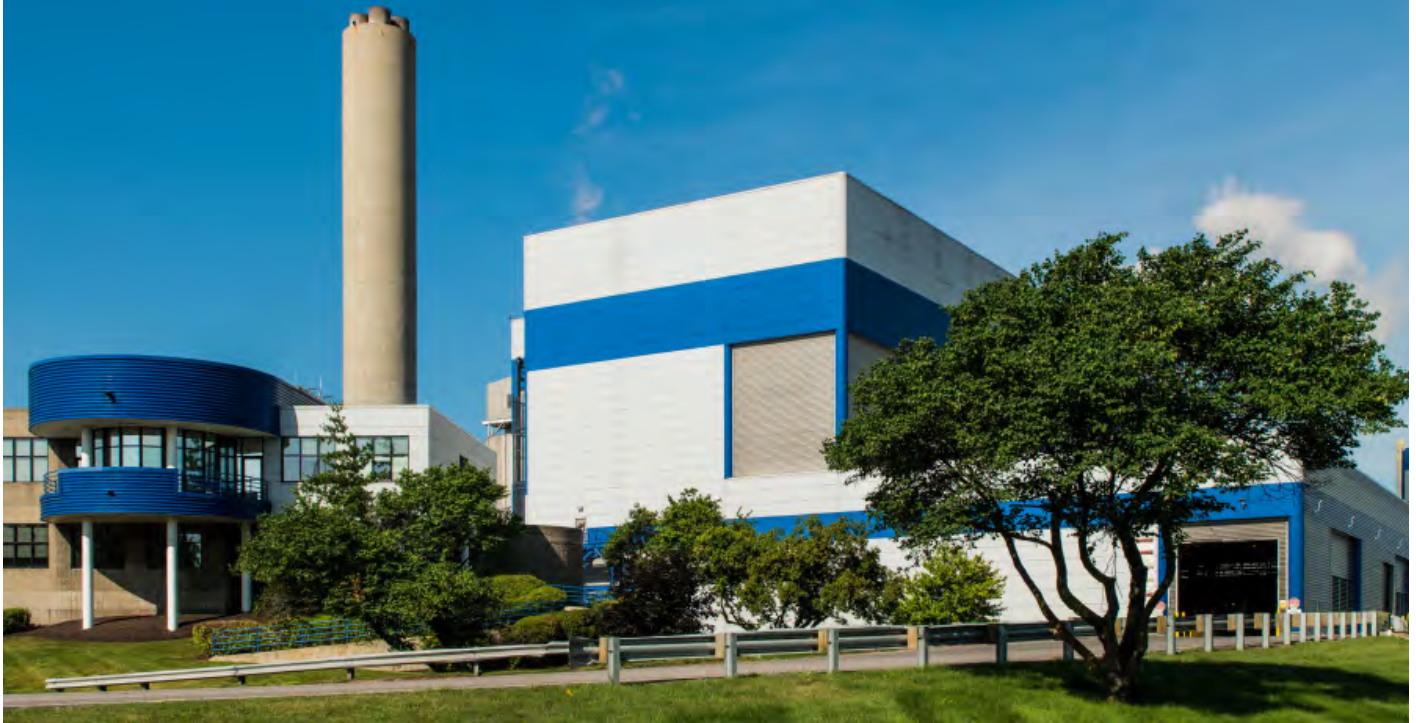
Covanta Indianapolis EfW facility
