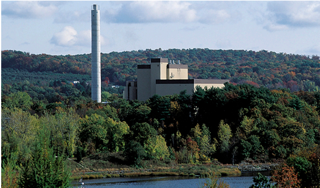
Covanta SECONN in Preston, Connecticut safely disposes of approximately 690 tons of municipal solid waste a day while producing 18.4 MW of renewable energy.
