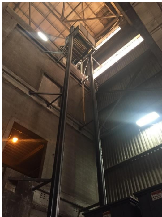
Figure 7 - WFS Elevator Unit to transport full & empty WFS bins
